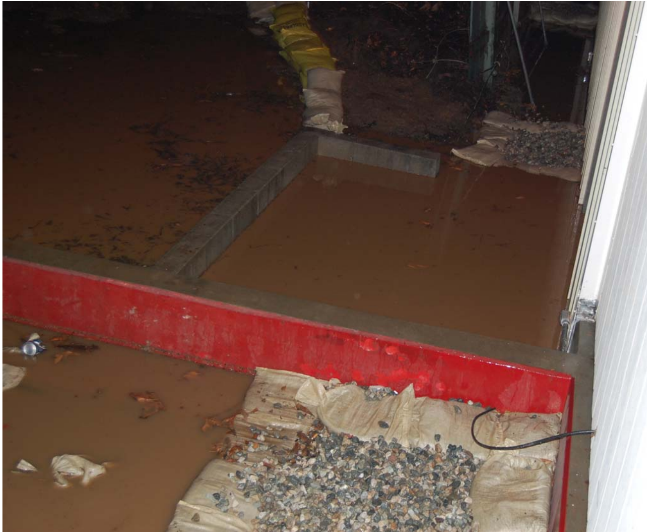
Someone thought it a good idea to block the drains on the building site to the North of the 40m.
